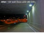
These photographs show a practical example of our energy efficient LED products in the field. We replaced 400 watt high pressure sodium tunnel fixtures with Esco LFL 120 watt tunnel fixtures.
